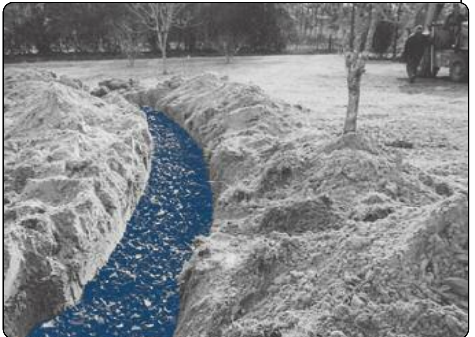
Pipe covered with two inches of tire chips.
